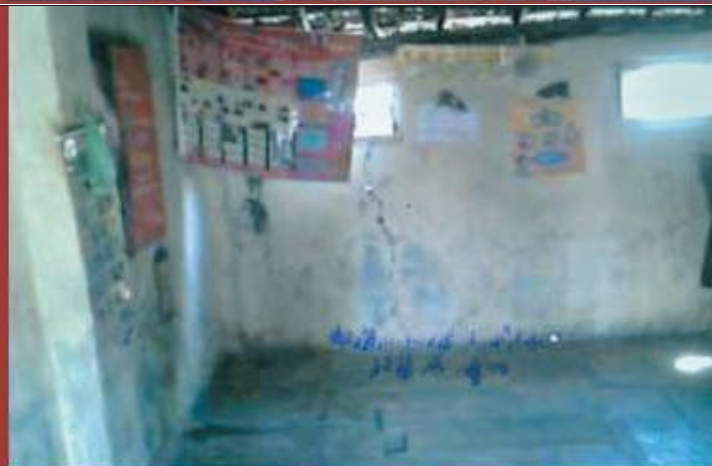
Exhibit 4.8 Umbhed-1 Anganwadi Centre, project Kamrej district Surat, Gujarat housed in a kachcha building
